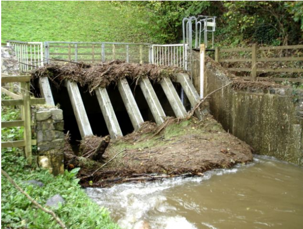
Figure 8.1 Coarse screen at a flood relief culvert inlet showing degree of debris build-up (the 'Beaverscreen' effect).
