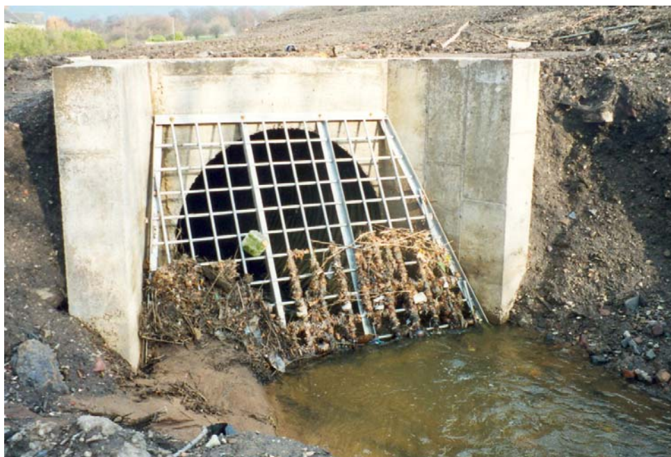
Figure 4.2 Poorly designed screen.
