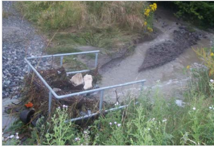
Figure 3: Upstream Trash Screen after the Flood
