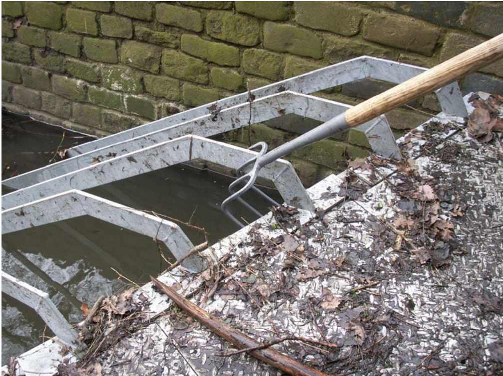
Figure 11.3 Trash screen in a public park.
