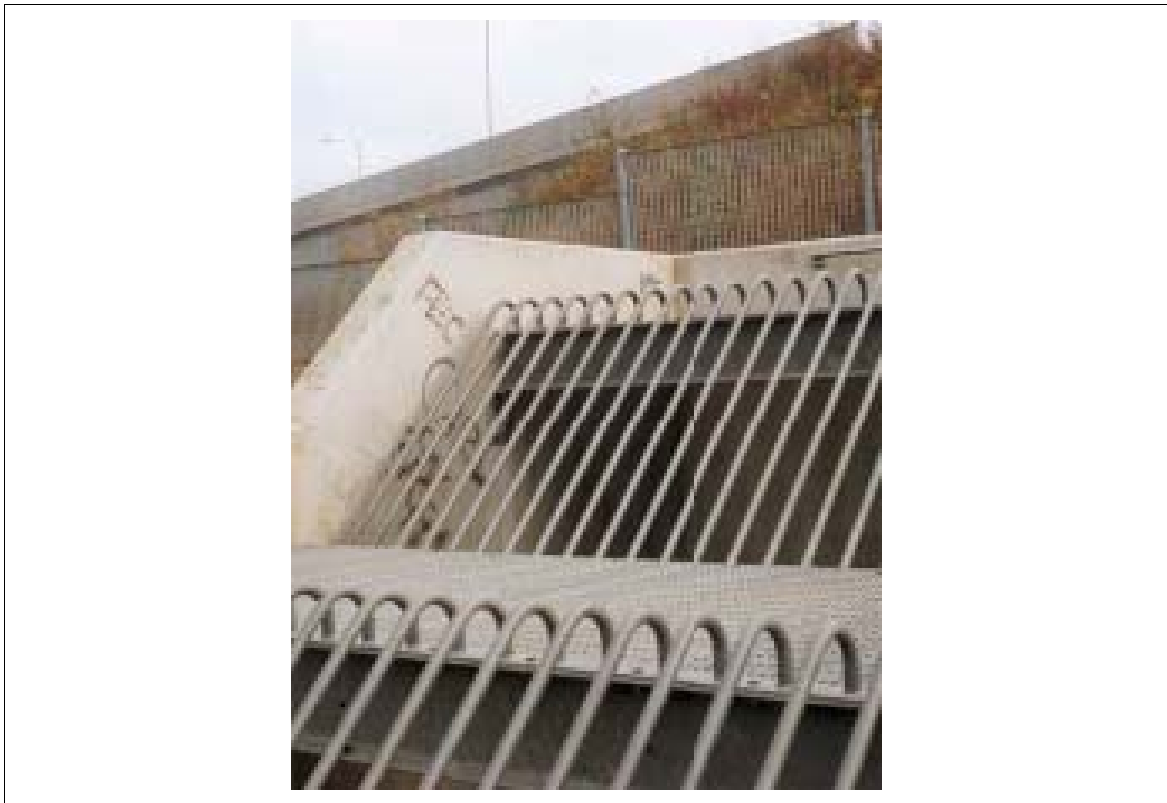
Figure 8.2 Design tolerances allowed children to squeeze between the concrete sidewall and the end bar on the screen.
