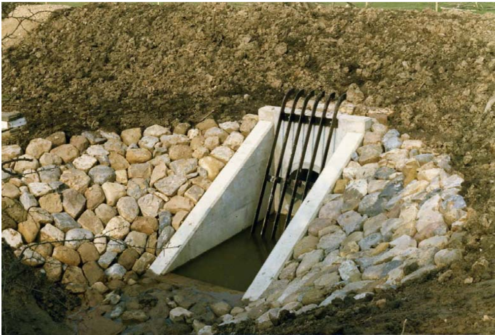
Figure 11.2 A debris screen on a small culvert.
