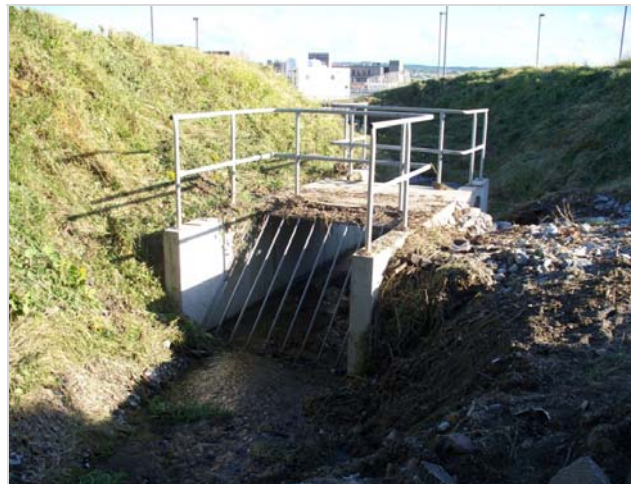
Figure 1: Upstream Trash Screen
