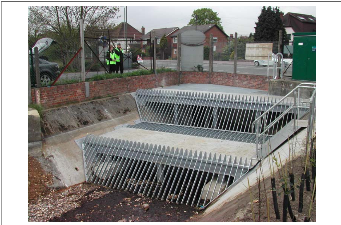
Figure 11.1 A recently installed screen in an urban setting.
