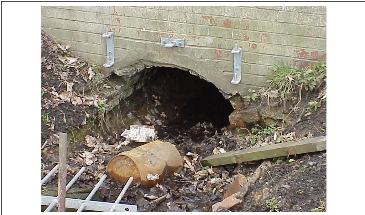
Figure 4.3 Screen on a small culvert not securely fixed in place.
