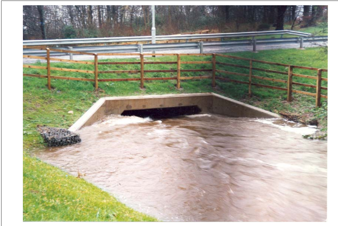
Figure 3.1 Highway culvert with no requirements for a screen.
