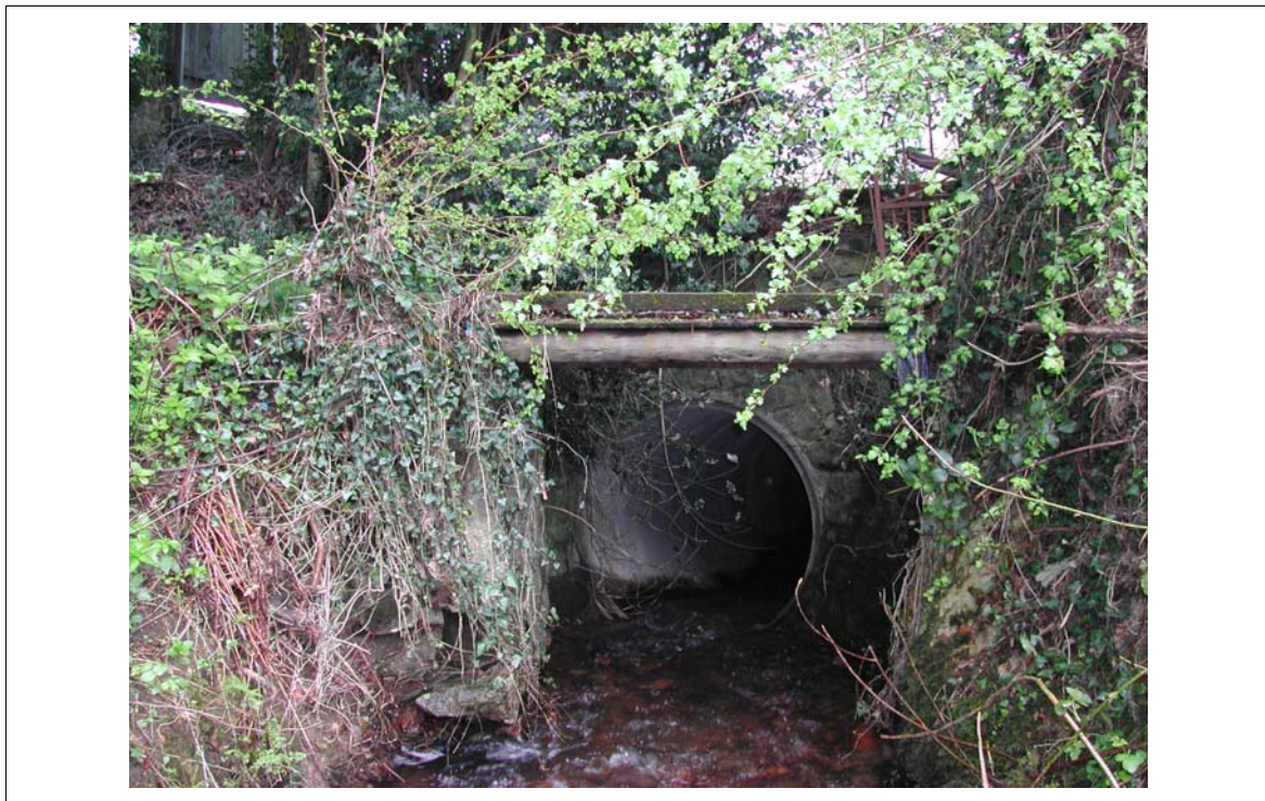
Figure 4.1 Culvert inlet on private land.
