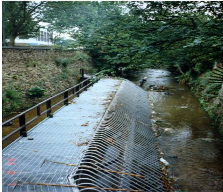
Figure 11.4 Screen on the River Sheaf with diagonal alignment to flow.
