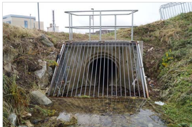
Figure 2: Downstream Security Screen
