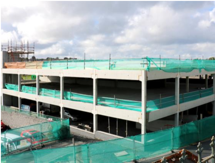
Construction site for new multi-story car park at University Hospital Galway, taken on the 27th of August 2015
