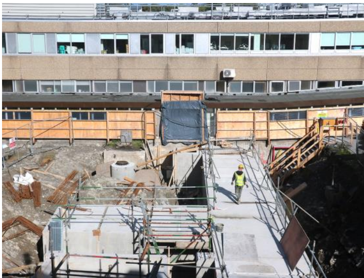
Construction site for new ward block at University Hospital Galway, taken on the 27th of August 2015
