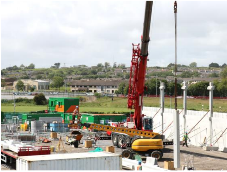
Construction site for new multi-story car park at University Hospital Galway
