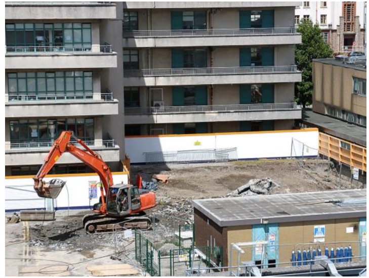
Construction site for new ward block at University Hospital Galway
