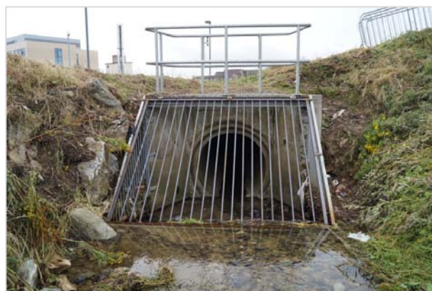
Figure 2: Downstream Security Screen (replacement screen)
