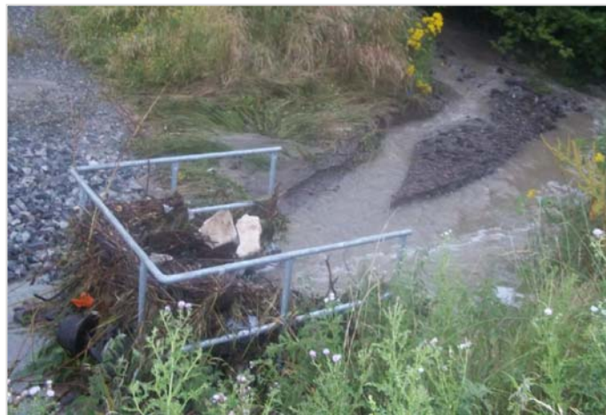
Figure 3: Upstream Trash Screen after the Flood
