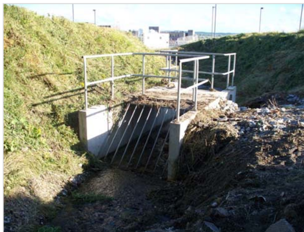
Figure 1: Upstream Trash Screen
