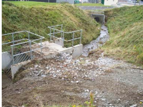
Figure 2: Screens and Culvert Entrance (photo taken 30th July 2013)
